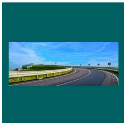
W Beam Metal Crash Barrier
